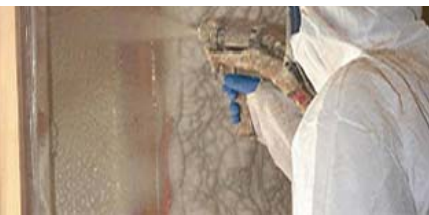
SPF spray application on wall
